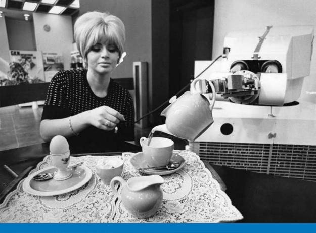
In a 1960s demonstration, a Unimate robot poured a cup of tea to show off its abilities.
